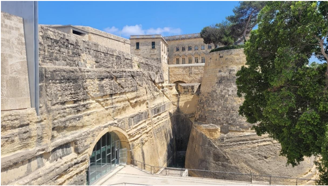
Figure 1- Valletta, Old railway train station
