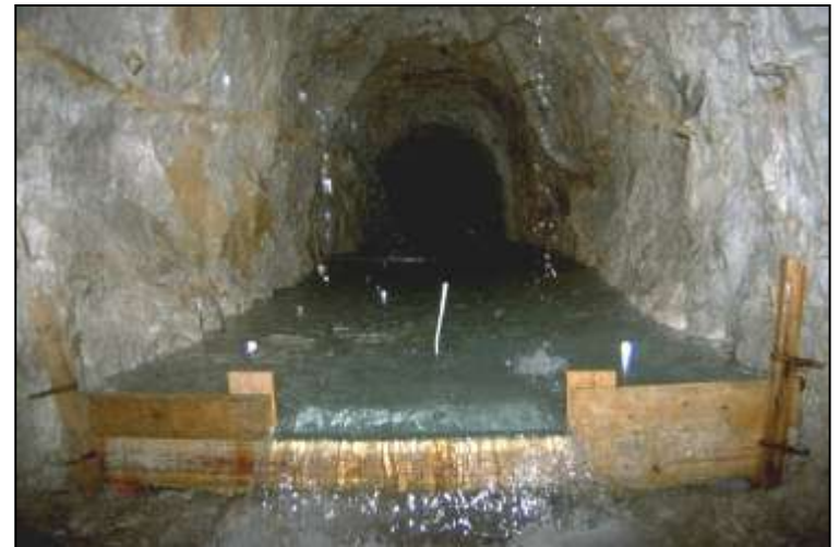
Drinking water drainage gallery in an alpine karst aquifer
